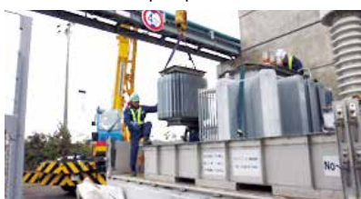
Treatment of PCB waste
