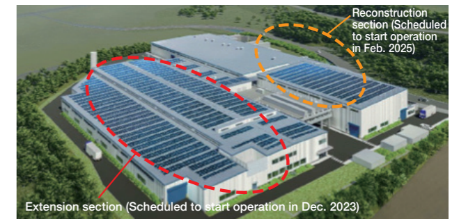
Seto Plant (Image after construction of new building)
