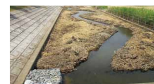
Waterway after dredging
