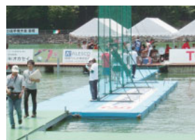
Floating dock installed
