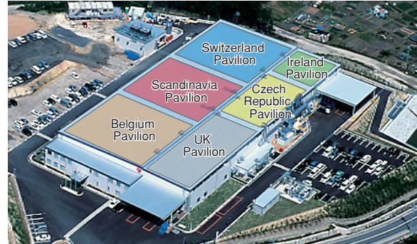
■ The 6 pavilions whose steel was reused to build the Seto Plant
