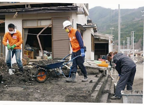
"Sludge Removal Action" by employees
