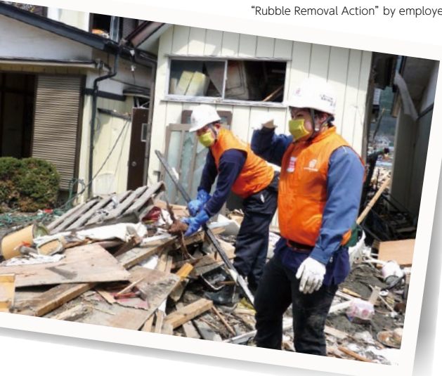
"Rubble Removal Action" by employees
