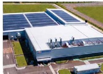
New Miyagi Ohira Plant
