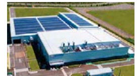
New Miyagi Ohira Plant
