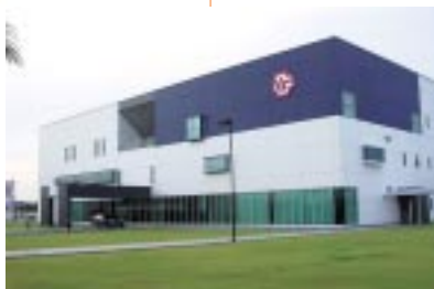
Toyoda Gosei Asia Co., Ltd., a management company for Southeast Asian operations, completed this new headquarters building in May 2004.
