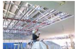
Ceiling reinforcement work
