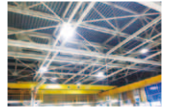
High-ceiling LED lighting
