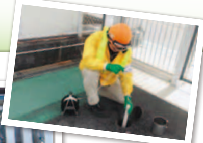
Groundwater inspection/ Haruhi Plant
