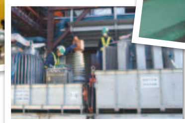
Removal of transformers containing PCBs/Inazawa Plant
