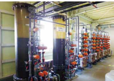
Wastewater treatment equipment / Inazawa Plant
