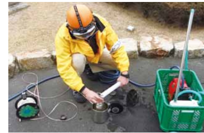
Groundwater inspection, Haruhi Plant
