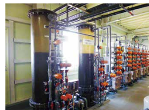
Waste water treatment equipment Drainage from plating processes is cleaned and reused in production
