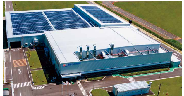
Toyota Gosei East Japan Co., Ltd. Miyagi Ohira Plant
